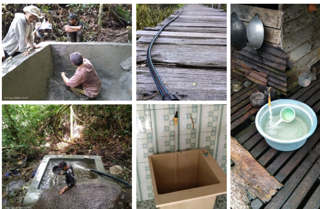
Fig.2. Development of clean water supplies installation in Pelaik hamlet: water reservoir (top and bottom left), pipe (top center), clean water flowing to bathroom (center bottom) and to the washing place in one of the biliks (right)
